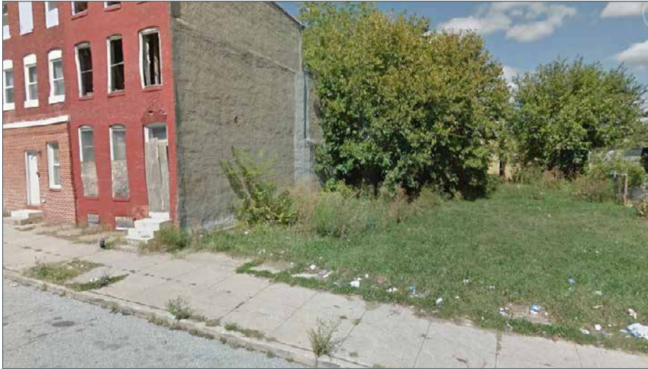
Figure III-20: Vacant Lot and Building Maintenance Challenges
