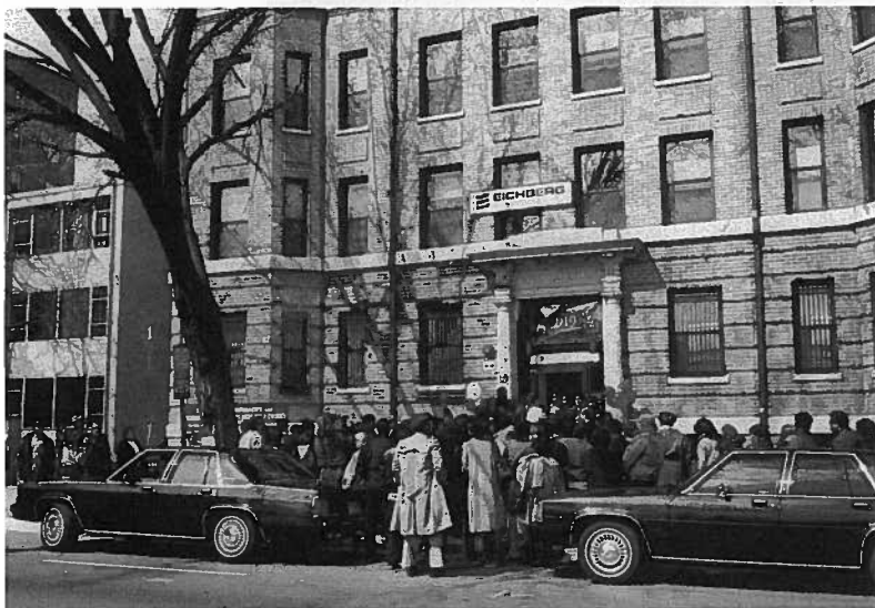
The 919 L Street Cooperative, before and after rehabilitation. Washington Inncery Self-Help Papers , Courtesy, D.C. Community Archives, Washingtoniana Division, DC Public Library
