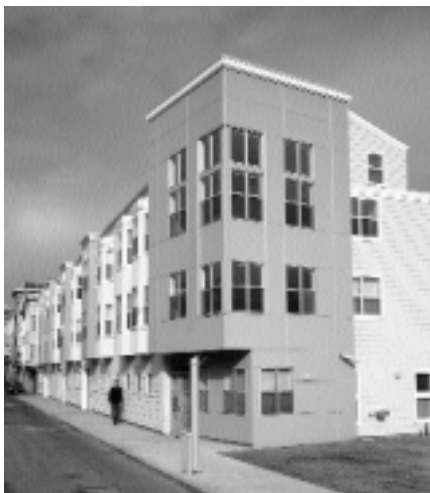
Minna Park Housing was recently completed by AND. Photo by Kevin Dwarka
