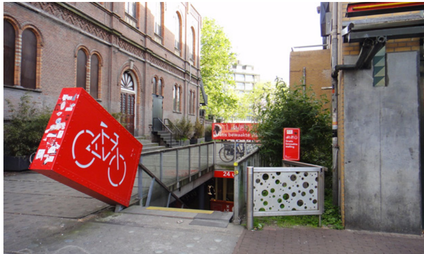
24-hour underground bicycle parking, near Leidseplein
