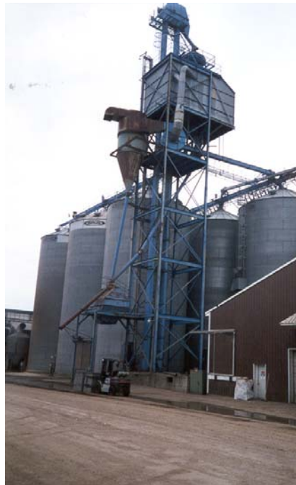
The Englevale plant
