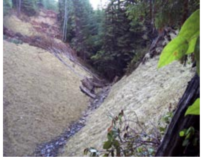
A sequence showing the decommissioning of a stream crossing. The original Humboldt crossing (logs laid lengthwise in stream and then covered with soil) had been overlain with a culvert. The entire crossing was excavated and approaching road segments decommissioned. Unstable fill on the road has been removed and the road was outsloped using the excavated spoil material. Mulching by hand prevents further erosion. Photo credit: Pacific Watershed Associates and the California Department of Fish and Game.
