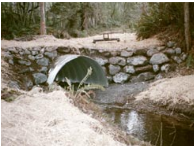
Replacing a culvert on the north fork of Widow White Creek to enable anadromous fish to access spawning habitat upstream. This project was a collaborative effort involving the McKinleyville Community Services District and Redwood Community Action Agency. Funding was provided by grants from the Department of Water Resources – Urban Streams Restoration Program and NOAA Fisheries Community-based Restoration Program. Photo credit: Don Allan, Natural Resources Services, RCAA.
