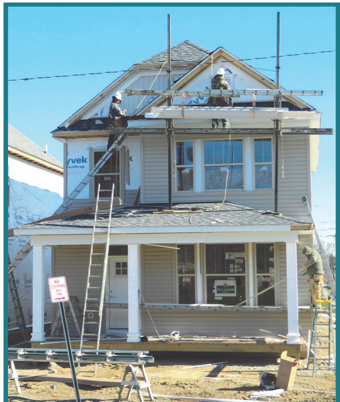
Wagenbrenner Development Company home under construction at Hamlet St. & 8th Ave.
