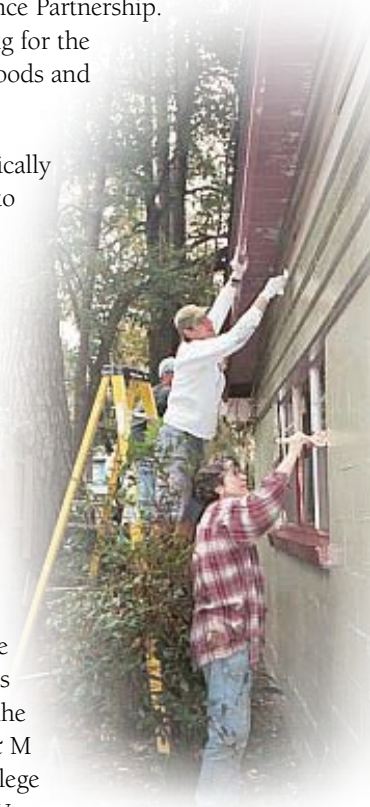
Volunteers fix and paint a resident's home, while others work on the yard.
