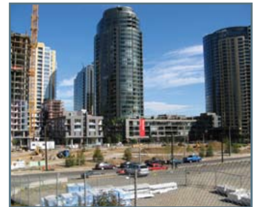
Redevelopment is underway at Portland, Oregon's South Waterfront
