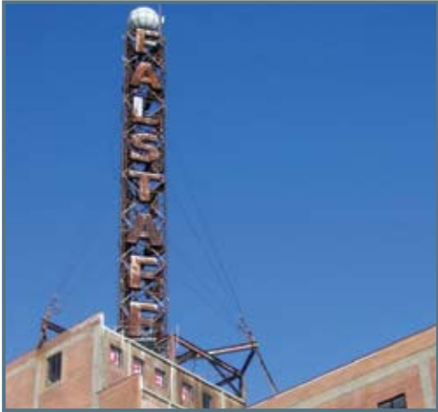
The weather beacon atop Falstaff's tower provided local weather forecasts by using colored and flashing lights
