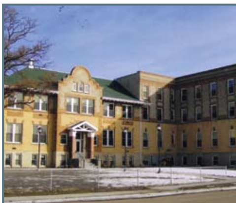
Using EPA and HUD funding, a deteriorating building in Miles City, Montana was transformed into affordable housing
