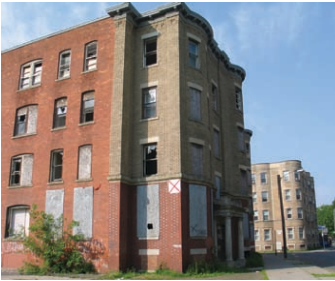
The City of Springfield has slated several properties in its South End neighborhood, where this vacant building is located, for priority redevelopment.
