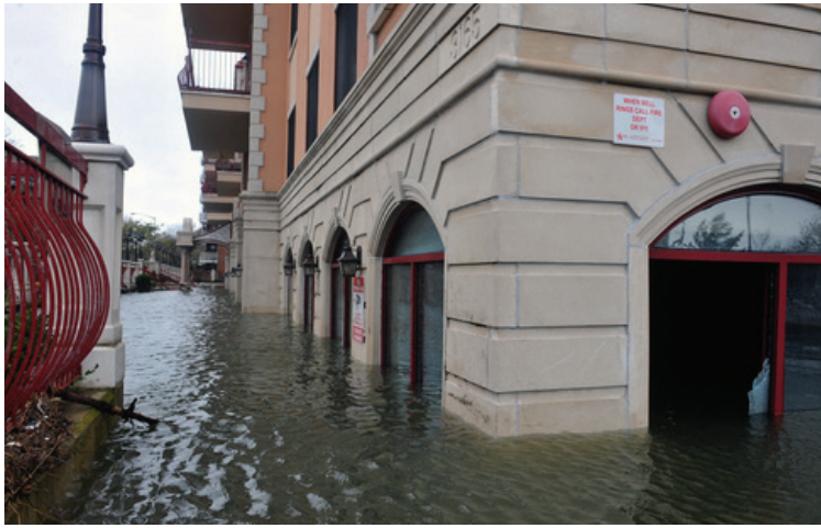
Flooding in Sheepshead Bay, Brooklyn.
