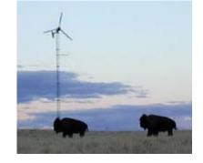
electric fences. Doug's 60-ft guyed turbine is interconnected to Glacier Electric Cooperative utility grid. Doug's turbine was originally installed during October 2003.
