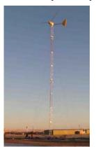
The Liberty County wind turbine is designed to offset electrical power used by the county's maintenance shop, as well as provide a working example of how wind power can benefit local government. The turbines sits atop a 100 ft tilt-up tower and interconnected to Northwestern Energy's distribution grid. The turbine was installed in December of 2003. County Commissioner, Don Marble, championed the installation and currently serves as OWC's Vice President.
