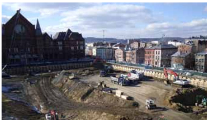
Washington Park – under construction. Source: Cincinnati Center City Development Corporation.
