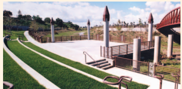
The 500-seat, outdoor amphitheater features a stage that rises and lowers with the water level of the creek.
