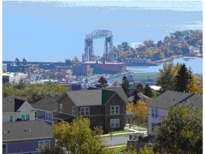
Harbor Highlands Phase II Current Construction – 42 new units + child care including 17 public housing replacement units
