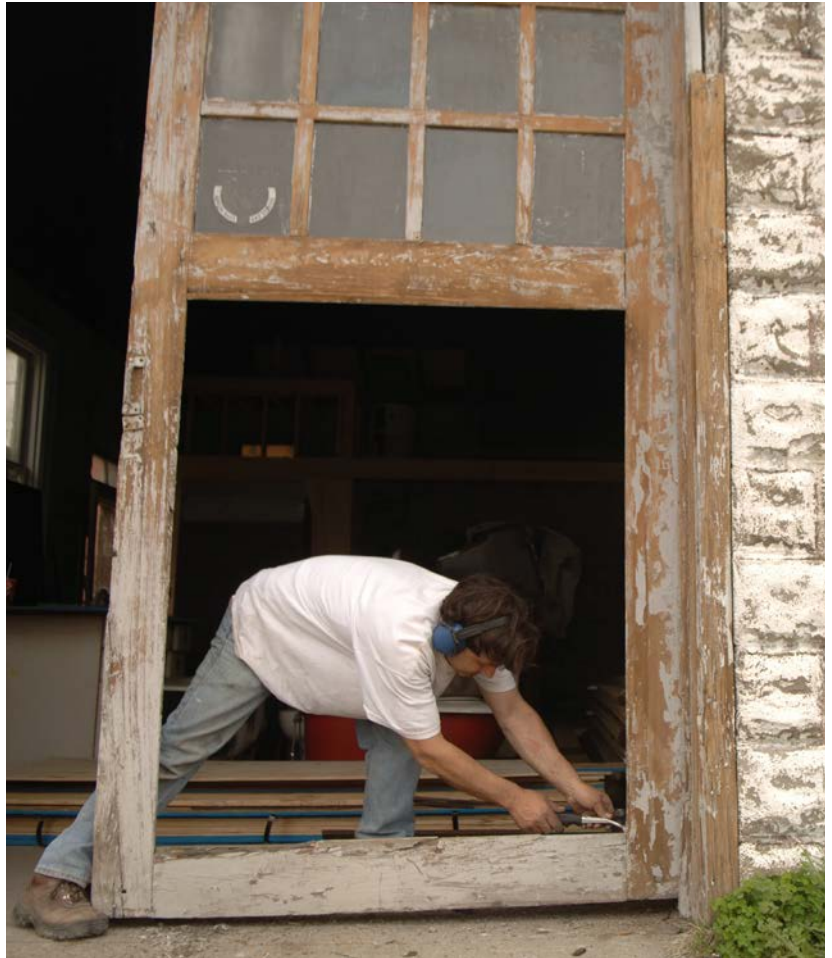
Above: Renovation of abandoned buildings in Southeast Indianapolis
