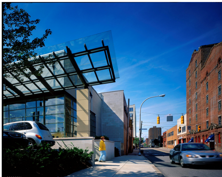
Entrance to Whole Foods parking lot, East Liberty, Pittsburgh
