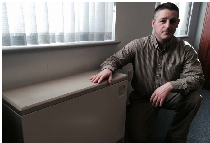
David Wood, CMLP's general manager, with a Steffes heater. The unit is full of ceramic blocks that are heated with electricity overnight and warm his office by day.
